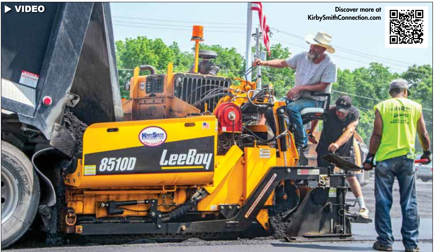
Supervisor Farin Deck operates a LeeBoy 8510D paver as J&B Asphalt & Paving lays down a new parking lot in Independence, Mo. "It's smooth and easy to operate," said Deck. "The push-button electric screed is great and gives us more even heating."
