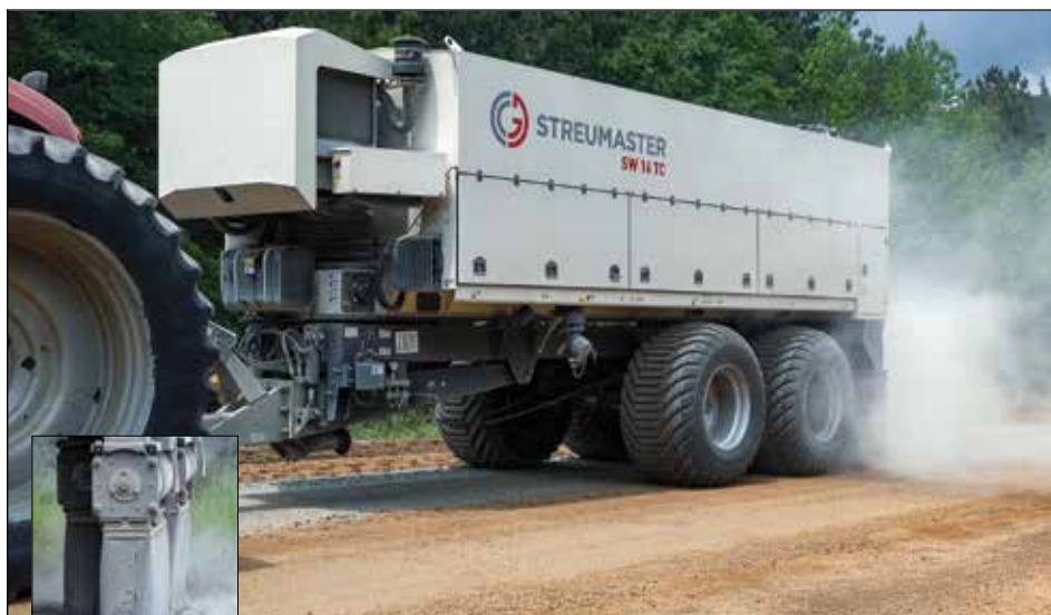
Before starting the full-depth reclamation with foamed bitumen process, a precise amount of cement is put down on the roadway with a Streumaster SW 16 TC binding-agent spreader.
