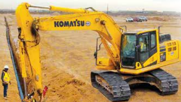
A Lockhart Excavation crew installs pipe with a Komatsu PC210LC-11 excavator on a subdivision in the Odessa, Texas, area. "The excavator is fast, so we can put pipe in quickly," said operator Raul Arellano.
