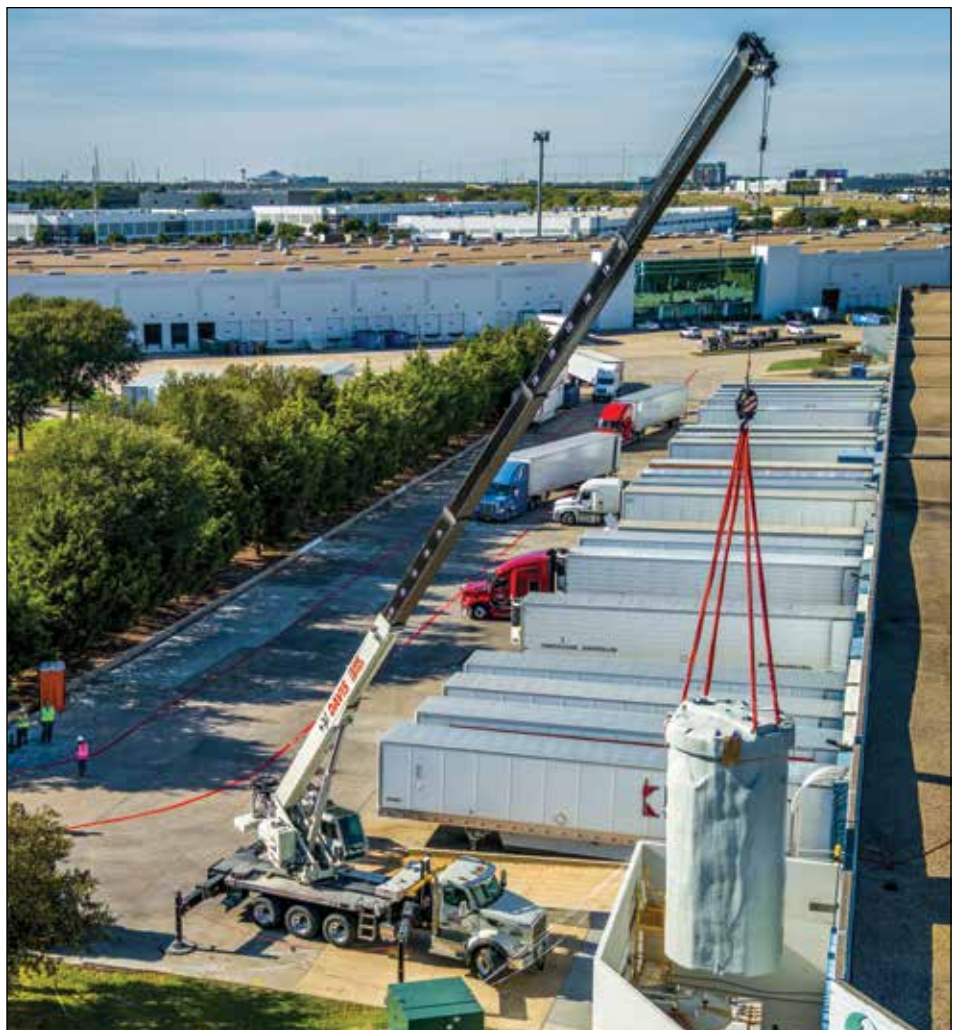
A Davis Crane Group operator lifts a tank part with a National Crane NBT60XL boom truck on a jobsite in the Dallas-Fort Worth area.
