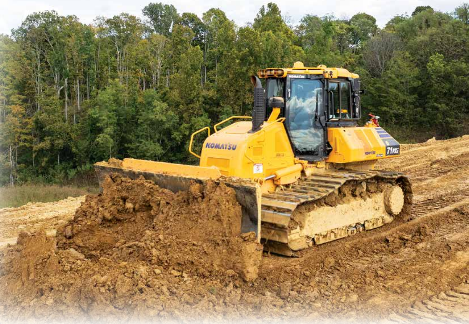
Implementing Komatsu Intelligent Machine Control (IMC) dozers and excavators is a good introductory step in adopting Smart Construction solutions.
