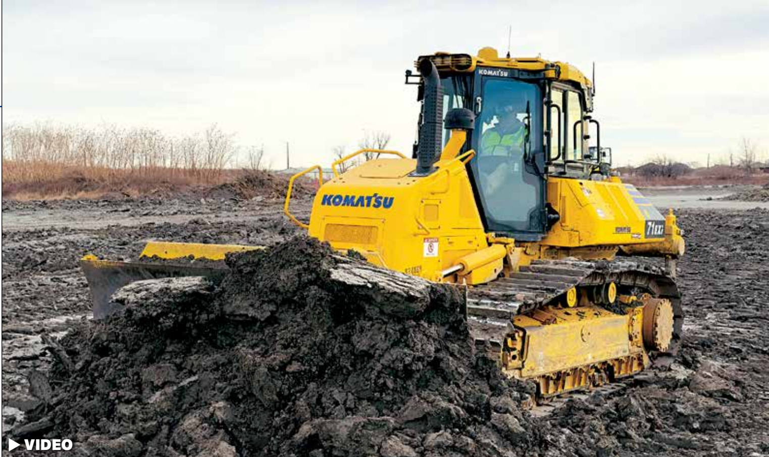
An L.A. Fuller and Sons operator builds a pond in Amarillo, Texas, with a Komatsu D71EXi-24 intelligent machine control (IMC) dozer.
