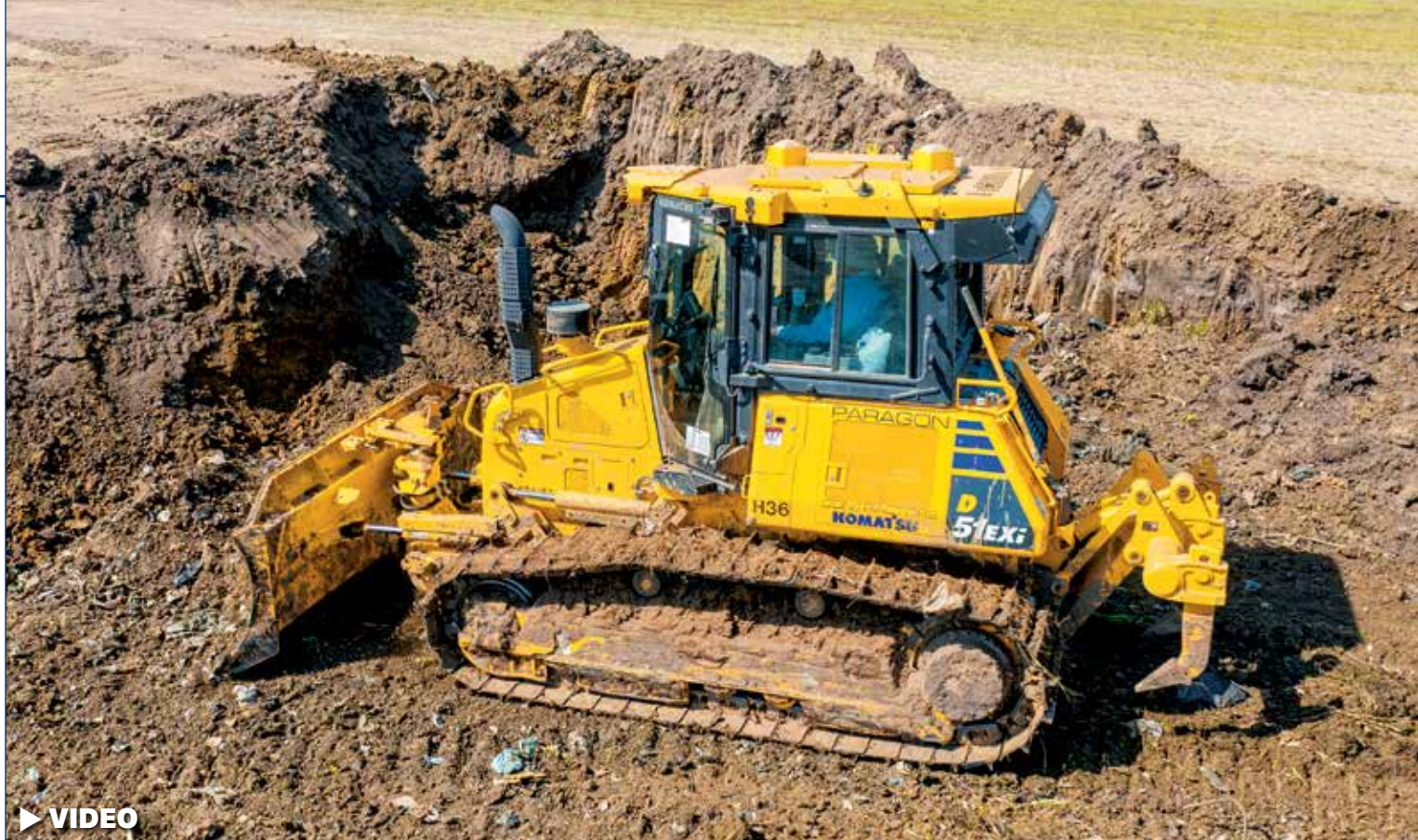
► VIDEO A Paragon Contractors operator grades with a Komatsu D51EXi IMC dozer.
