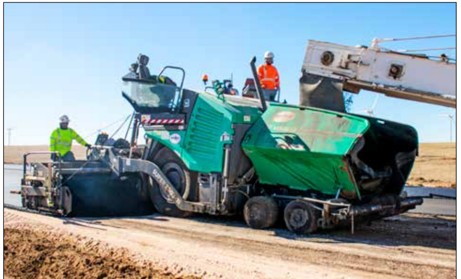
An L.A. Fuller and Sons crew paves an asphalt road with a VÖGELE SUPER 2003-3i paver and compacts it with HAMM smooth drum rollers.
